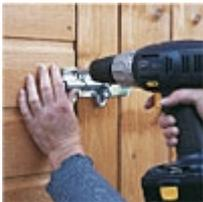
**4** Drill pilot holes and screw in the sliding bolt. This can be padlocked for additional security.
