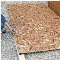
**6** Lay the roof panels on the ground, one at a time, with the eave sections (wooden strips) positioned underneath flush with the bottom edge of the panel. Measure and mark six evenly spaced fixing positions. Drill pilot holes and then hammer in the nails to attach the eave sections to the roof panels.
