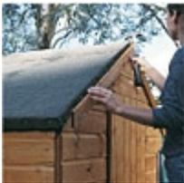
**3** Tidy up the felt at the corners: cut it to the edge, fold it neatly and tack it down. Hammer the roof fascia in place using 40mm nails over the felt on the front and back gable ends. Use four nails per strip.
