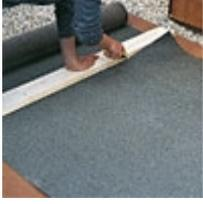
**1** Unroll the roofing felt then measure and cut three pieces: one for each roof panel, and a third strip to be laid along the apex, to prevent water seeping in. The pieces covering the roof panels should run the full length of the shed with a 50mm overhang at either end. The third piece covering the apex should be the same length and extend at least 75mm over each roof panel.
