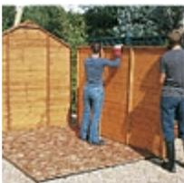
**2** Lift the gable end without the door into place, and use a prop to hold it upright. Lift one side panel onto the base.
