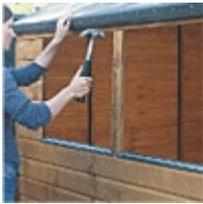
**2** Still outside, nail in the window cloaks (short strips of wood), using four 40mm nails in each. This secures the sills.
