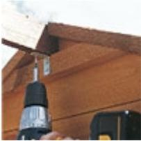
**5** Fit the roof support beam across the top of the shed, slotting it into the pre-cut grooves at the top of the gable ends. Check that the shed is sitting firmly on its base and that the door opens easily. Then use 30mm screws through an L-shaped metal bracket to fix the beam to each gable end.
