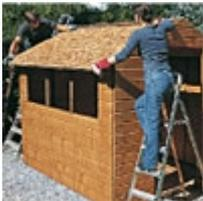
**7** Lift the roof panels into place one at a time. Line up the shed frame on the base using the centre markings then secure the roof panels with 30mm screws along the roof support beam. Fix them to the sides and gable ends of the shed using 40mm nails, or 30mm nails across the window heads. Check again that the shed is square on the base before finally nailing the sides and gable ends to the floor with 50mm nails.
