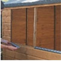
**1** Standing outside the shed, slot the metal window sill into position along the bottom of the window frame.
