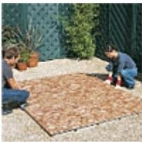
**1** Centre the shed floor on top of your concrete pad so that there is an overhang of 25mm on all sides. Measure and mark in pencil the centre point of each edge, and do the same on the bottom batten of each of the side panels.
