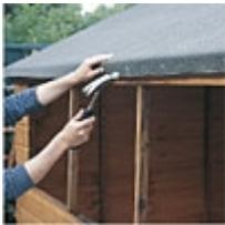
**2** Lay the first piece of felt over one side panel, with a 50mm overhang at the eave. Tack it along the top edge with felt nails about 300mm apart. Then fix it down along the gable ends and eave with felt nails at 100mm intervals. Repeat the other side. Place the third strip of felt over the top of the roof and nail it along each edge at 100mm intervals.
