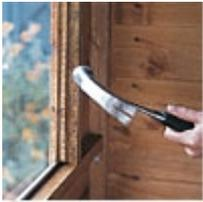
**3** From inside the shed, slide the perspex into place, resting it on the sill. The beading is secured with 25mm nails. Start the nails first, then position the beading over the perspex sheet at the top and sides of the frame and hammer them fully home. Finally remove the protective film from the perspex.
