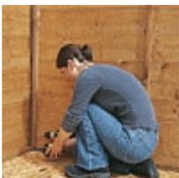
**3** Screw the gable end and side panel together along the framing battens where they meet. Drill pilot holes then fit three 50mm countersunk screws at the top, middle and bottom.
