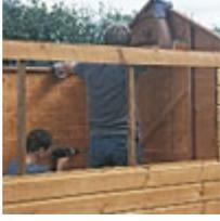
**4** Fit the other side panel in the same way. Then fit the gable end housing the door. But don't try to fix your shed frame to the floor yet.
