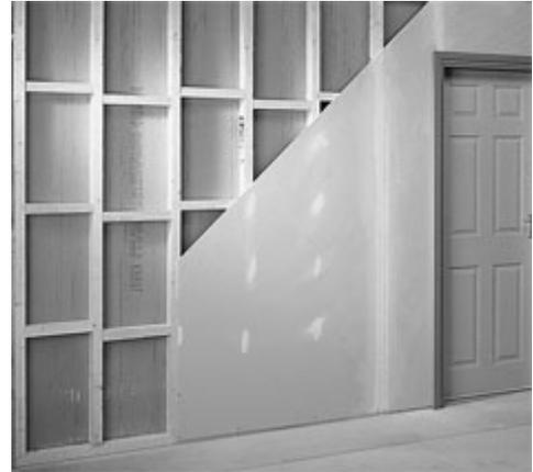
between studs for rigidity and for the fixing of heavy wall mounted items such as
